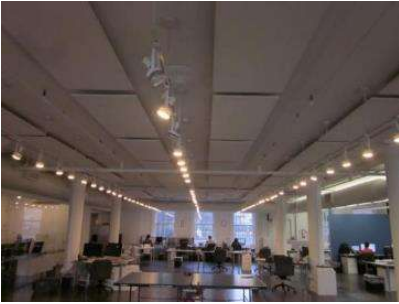
Dozens of bright point sources are used to provide general illumination to make room for acoustic panels
