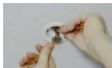
2. Press the escutcheon into place until secured
